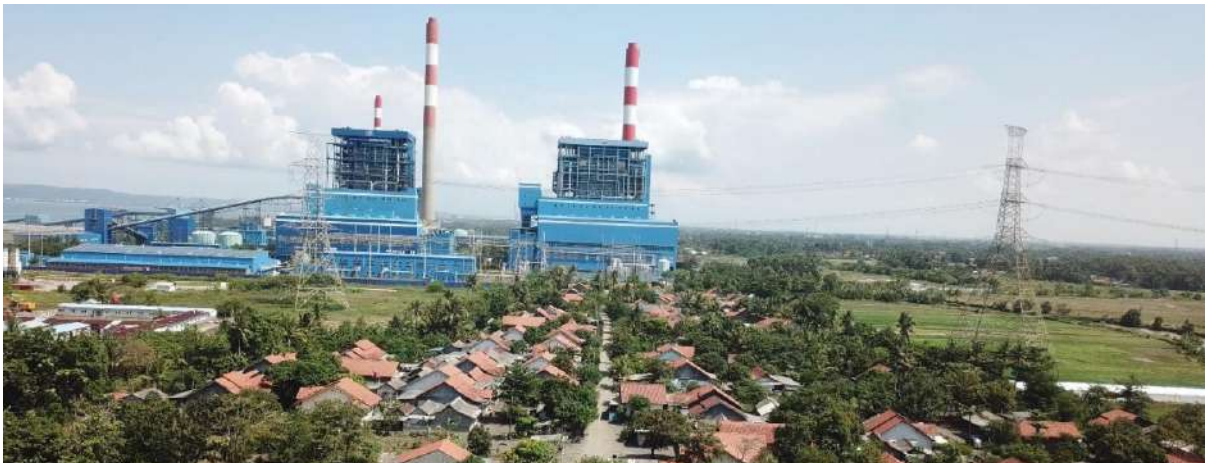
Ring 1 Karangandri Power Plant, Cilacap Regency, Central Java. Photo: CELIOS 2023
