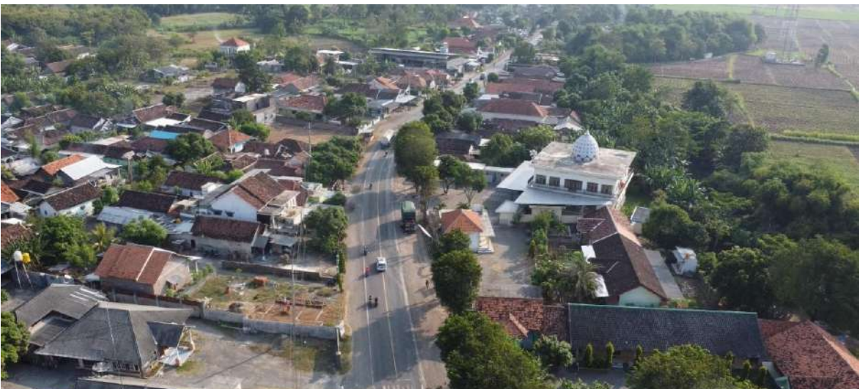
Ring 1 Paiton Power Plant in Jalan Raya Surabaya-Situbondo. There are no significant differences in the demographics and economic activities of the population compared to other areas along Jalan Raya Pantura.
